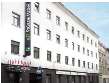
eFi Palace Hotel ***, Brno
